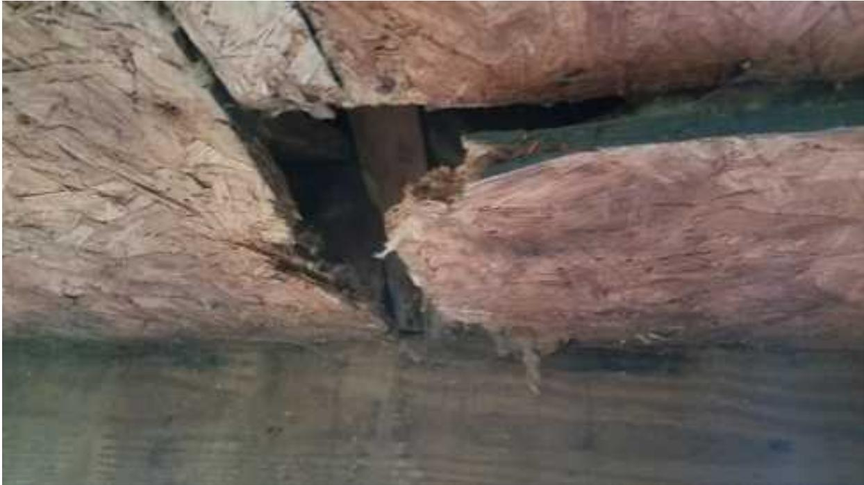
[2C.10](#) Wood: "First" wood untreated, too close to earth (8" or less) is prone to rot carpenter ant and especially termite damage as discussed. Repair/treatment is recommended to deter/stop termite activity
